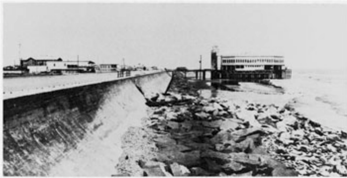
Figure 1 - The Galveston seawall. Note absence of beach. Photograph by W.T. Lee, USGS Photo Library, Denver, CO.
