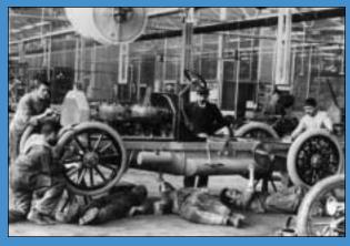
This photo, taken in 1904 inside Daimler Motor Co., is an example of the use of small-batch production, a production system in which small groups of people work together and perform all the tasks needed to assemble a product.
