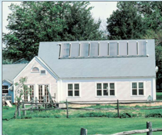
The array of solar cells of the roof of this house provides it with electric energy.
