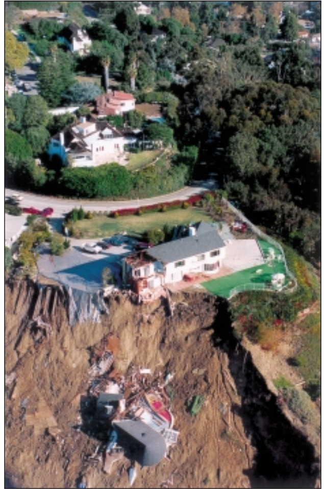
FIGURE 11.19 Parts of an expensive house slide down the hillside in Pacific Palisades, CA. Building at the edge of steep slopes made of unconsolidated sediment in an earthquake-prone region is a risky venture.
