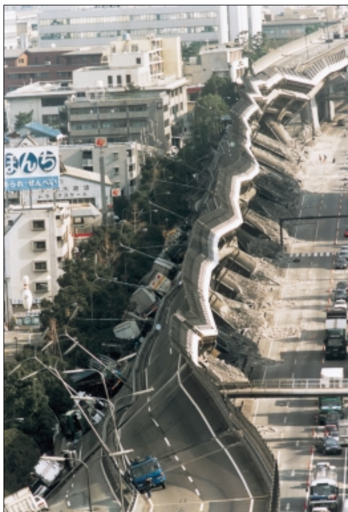
FIGURE 11.15 An elevated freeway buckled and collapsed as a result of the 1995 earthquake in Kobe, Japan.
