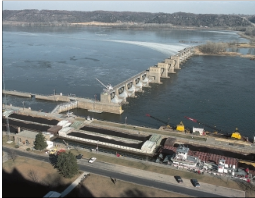
FIGURE 11.18 Locks, dams, levees, and other flood control and navigational structures such as this complex on the Mississippi River at Dubuque, IA, have been a godsend for commercial shippers but have also been disastrous for riparian ecosystems, backwater sloughs, marshes, and the wildlife that depends on them.
