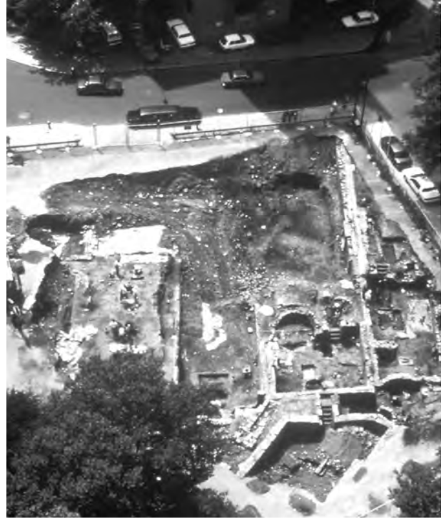
FIGURE 1.5 Excavations on the site of a new courthouse at Foley Square in lower Manhattan exposed the remains of tenements that were part of the infamous Five Points neighborhood. The excavation was done by Historic Conservation and Interpretation (HCI) in 1991; artifact analysis and interpretation were completed by John Milner Associates under contract to the U.S. General Services Administration.
