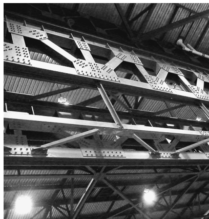
Photo 4.1: Massive roof trusses with bolted joints and gusset plates.
