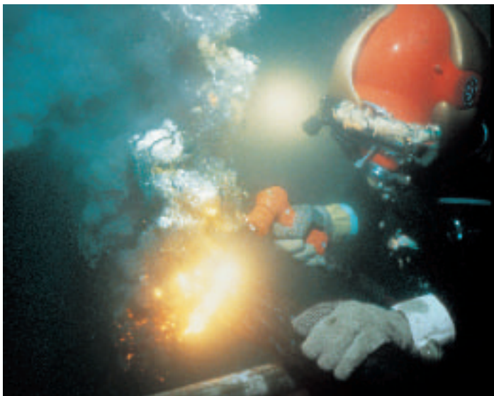
Figure 6 This welding torch burns hydrogen and oxygen to produce temperatures above 3,000°C. It can even be used underwater.
