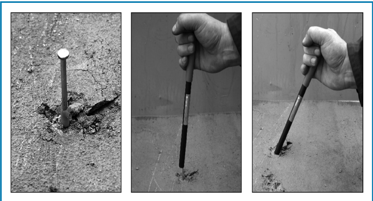
Fig. 17.16 Safe nail removal
