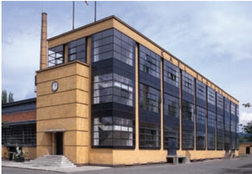
Walter Gropius, the Fagus Factory Completed in 1913, this innovative factory building displayed architect Walter Gropius's desire to remove decorative clutter and to allow natural light to penetrate to the structure's interior.
