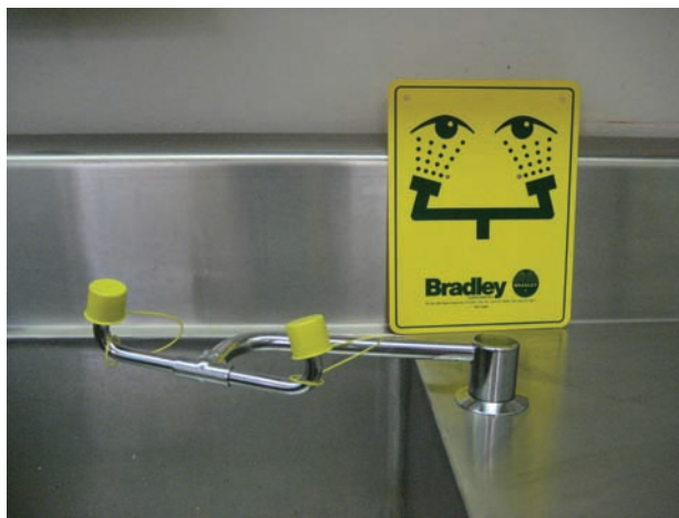
Figure 1-11 An eyewash station is an instant source of water for a quick rinse when an accident occurs. A quick response can be crucial.
